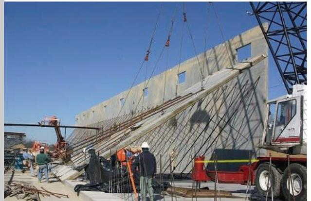
An example of a tilt up panel being raised into place
